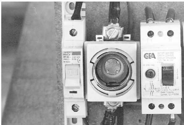
Fig. 4.21 Earth leakage circuit breaker
